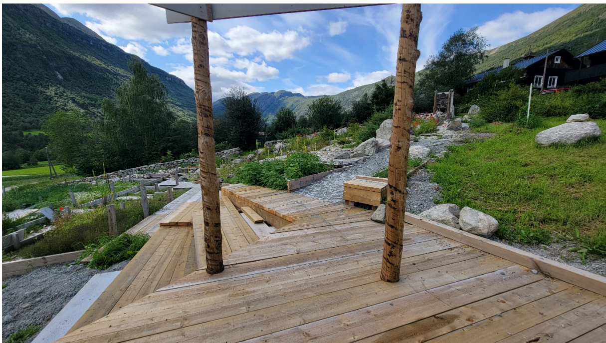
... and landscape temple under construction!
